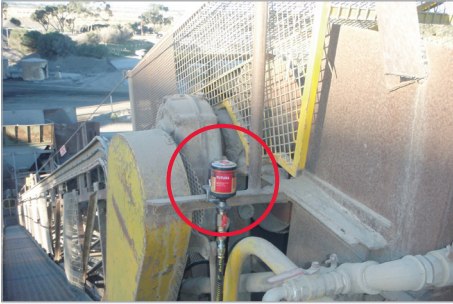
Lubrication of pillow block on a pressure pulley
